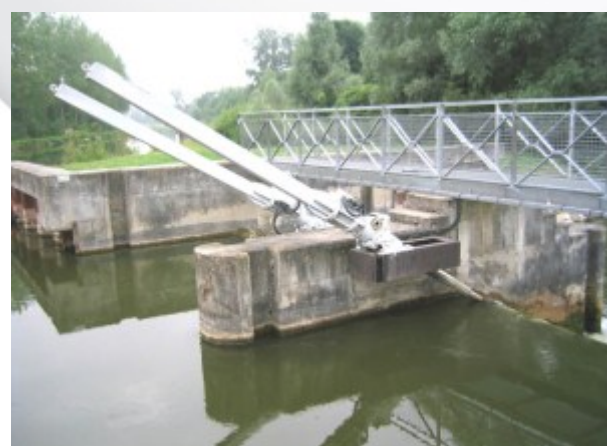
Mechanical jack on weir gate
