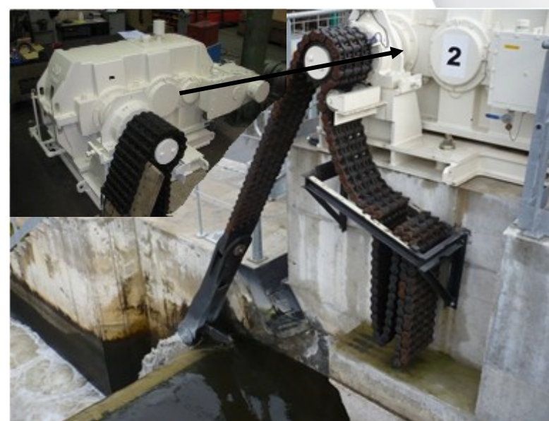
Helical drive unit - pinion - chain - monitoring
